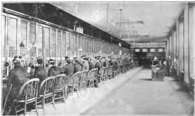
TELEPHONE OPERATING OR SWITCH-ROOM, ON CORTLANDT ST., METROPOLITAN TELEPHONE AND TELEGRAPH CO.
